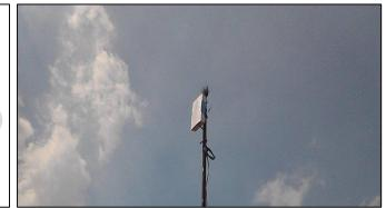
On base station side, a WBS is usually installed using a special bracket or signal tower due to the large size of the Sector Antenna. The Pharos Sector Antenna is designed with a dedicated slot to affix a WBS. You should fix the antenna to the signal tower with a metal bracket. For detailed information, please refer to the <u>TL-ANT5819MS Installation Guide</u>.
